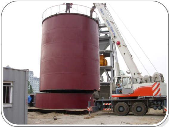
SILO CELL WELDING WORK
