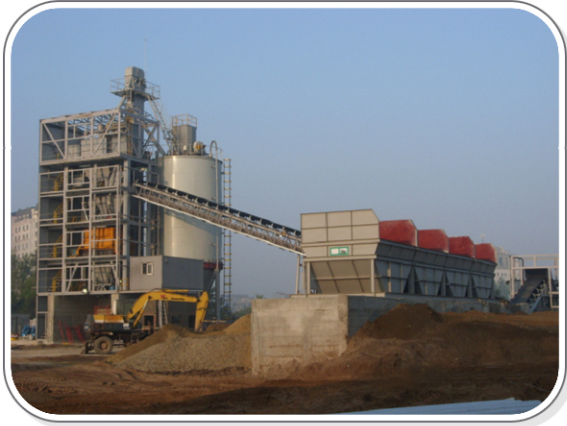
500TON Silo INSTALLATION
