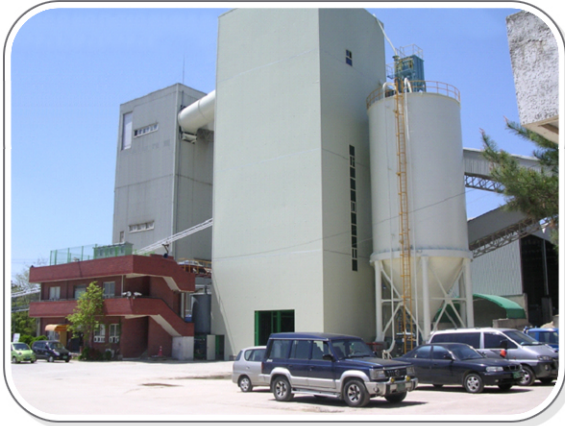
210M3/HR TOWER B.PLANT-KOREA
