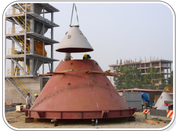
SILO CONE WELDING
